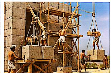
Ramps, pulleys, and scaffolding
