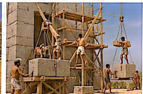
Ramps, pulleys, and scaffolding
