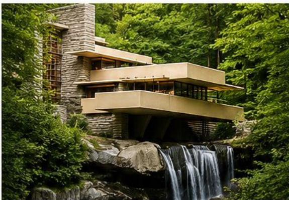
Fallingwater (USA) a house built over a waterfall.
