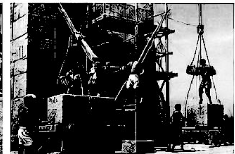
Ramps, pulleys, and scaffolding
